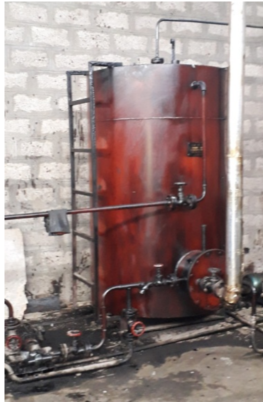
Not pre-heated Burner Oil
