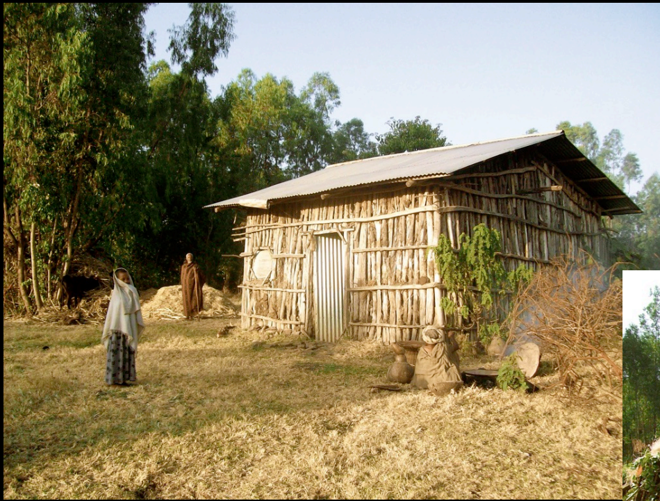
Existing traditional house construction and domestic life in Bura area
